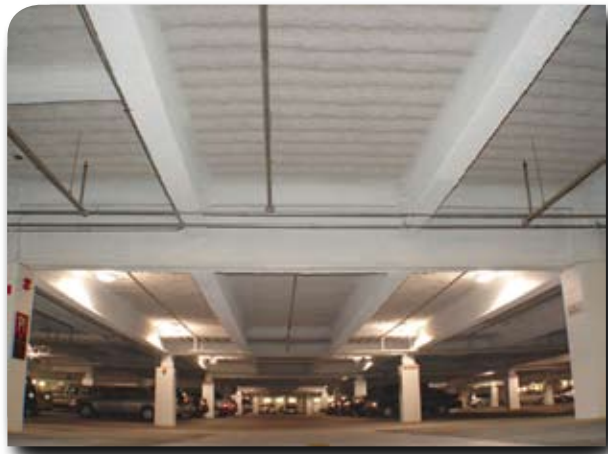
Boston University Arena (Boston, MA) K-13 Light Gray | 190,900 Square Feet | 3.4" Thickness
