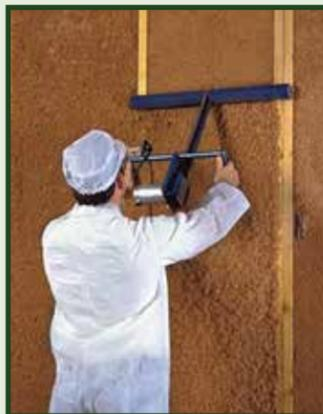
**STEP ONE:** A unique spray application that fully insulates around plumbing and wiring, reducing air infiltration and creating a comfortable environment.
